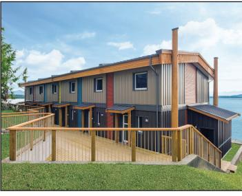
"Using off-site modular wood construction in a remote northern location resulted in limited on-site waste for a significant reduction in its environmental impact. The prefabricated wood design could be easily replicated across Canada. Wood plays an important role in obtaining Passive House standards."
