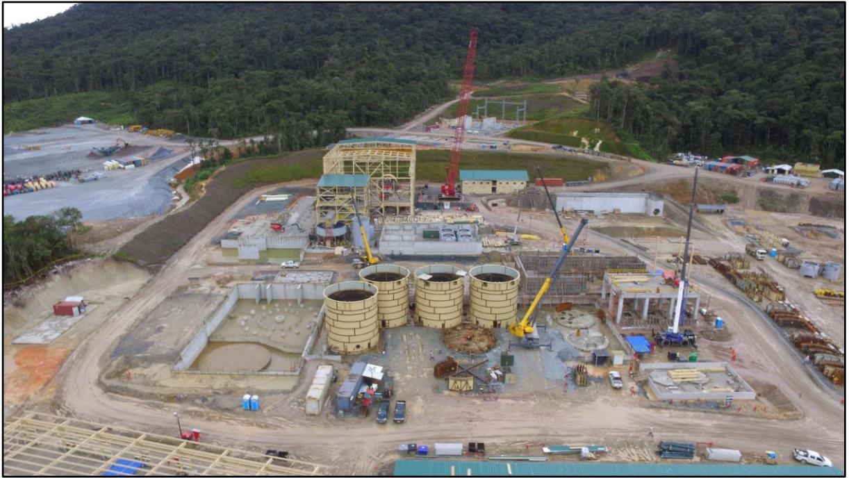
Figure 3. Process plant concrete 62% complete and steel erection 18% complete
