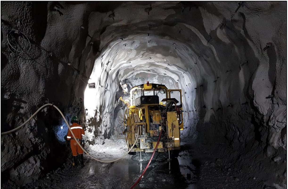
Figure 2. The declines have reached the orebody - development on primary levels underway
