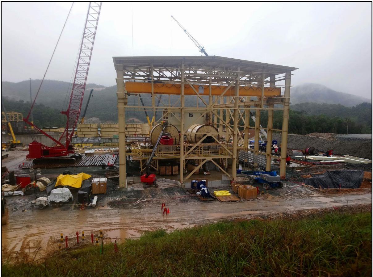
Figure 4. Process plant mechanical equipment - grinding mills and carbon-in-leach tank - installation underway
