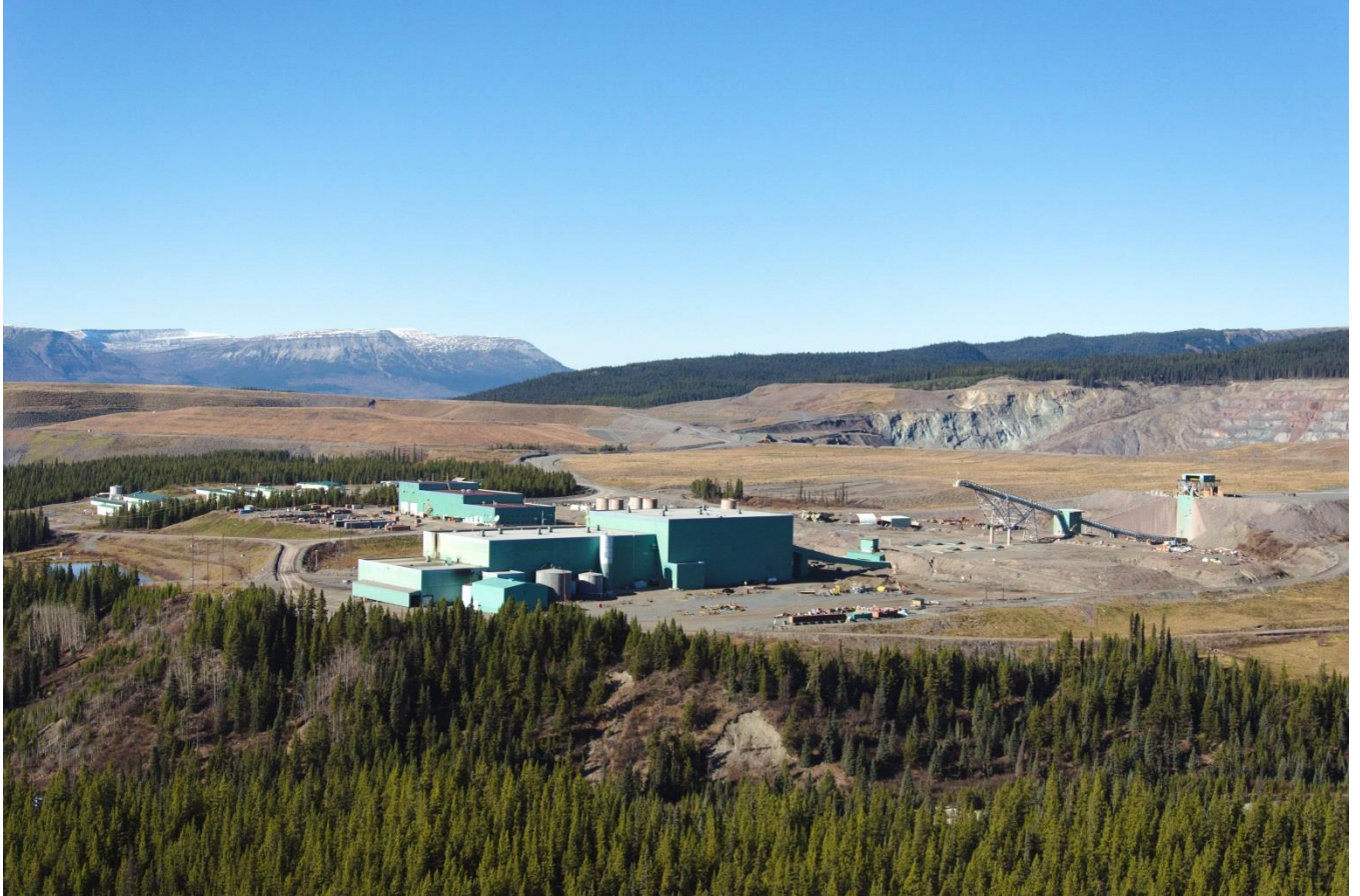
Appendix 1: Kemess Site (2015) showing processing facility (front), maintenance-administration facility and camp
