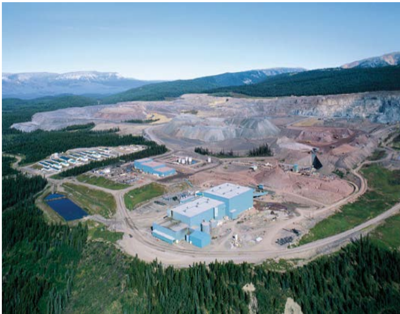
Figure 2: Kemess Property: Mill Processing Facility & Associated Surface Infrastructure
